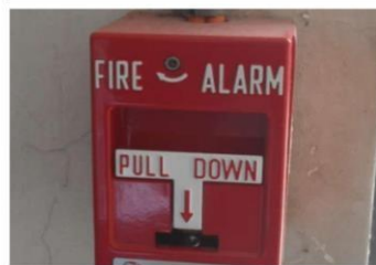
Fire Alarm Switch for Addressable Fire Detection System
